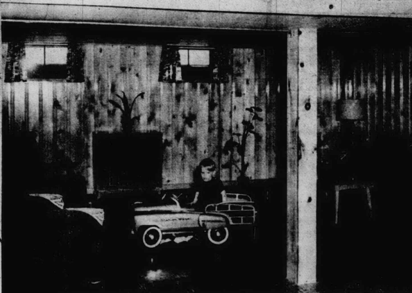
THE BASEMENT RECREATION ROOM in the home of John Downing of 1133 South Harvey street was finished by Downing himself, who spent his days off and evenings for six weeks working on the project. The walls are paneled in seven inch knotty pine boards, and the room features an acoustical ceiling. Downing also laid asphalt tiling on the floor in a design of light grey, red and ebony. The Downing home was recently constructed by Stewart Oldford and Sons.
