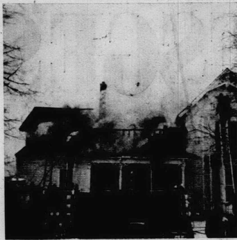
Roof falls, all blamed on faulty wiring
