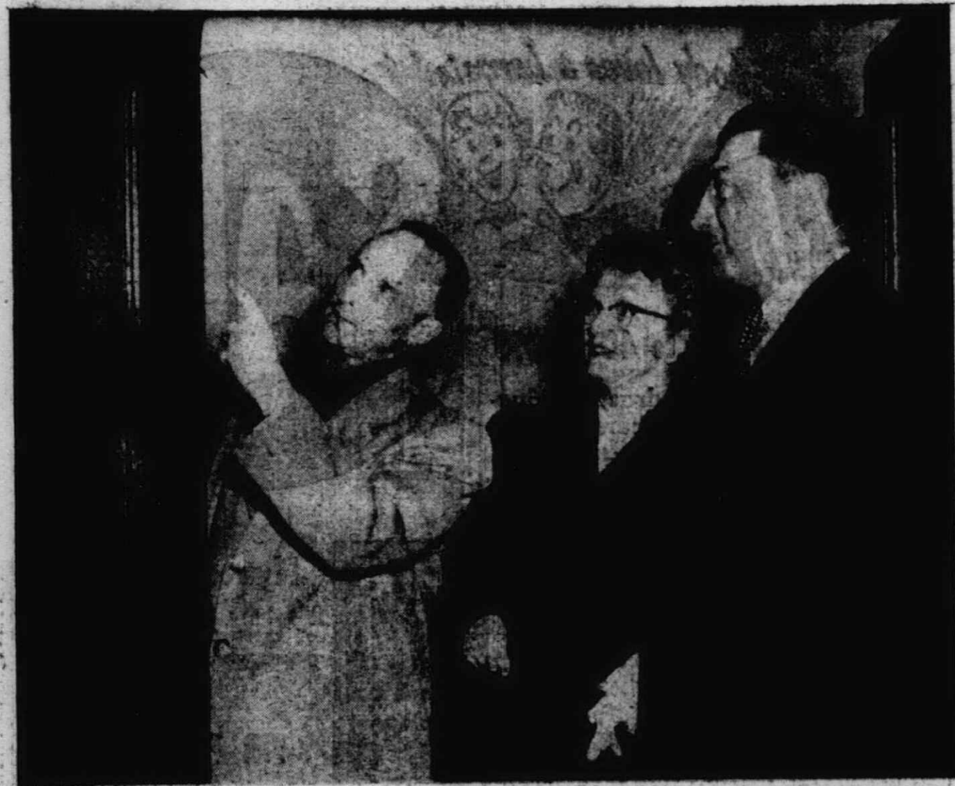
SAFEST FOR FIRES is the type of doors used by the Mayflower hotel, according to the inspection report made recently by insurance company fire inspectors who invaded the city. Checking the door is Frank Westerman (left), secretary of the Michigan Fire Protection association. Mrs. Florence Wood, local insurance agent, and Ralph Lorenz, hotel manager, happily hear the praising report of the hotel. (Ply-Mail photo)
