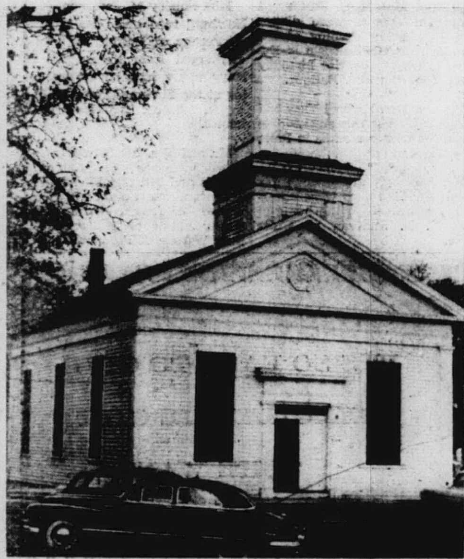
WEST SALEM COUNTRY church opened its doors three years ago after 15 years of emptiness except of Memorial day services. Reverend Patrick Clifford of Plymouth took on the reopening project shortly after he arrived in Plymouth to pastor Calvary Baptist church.
