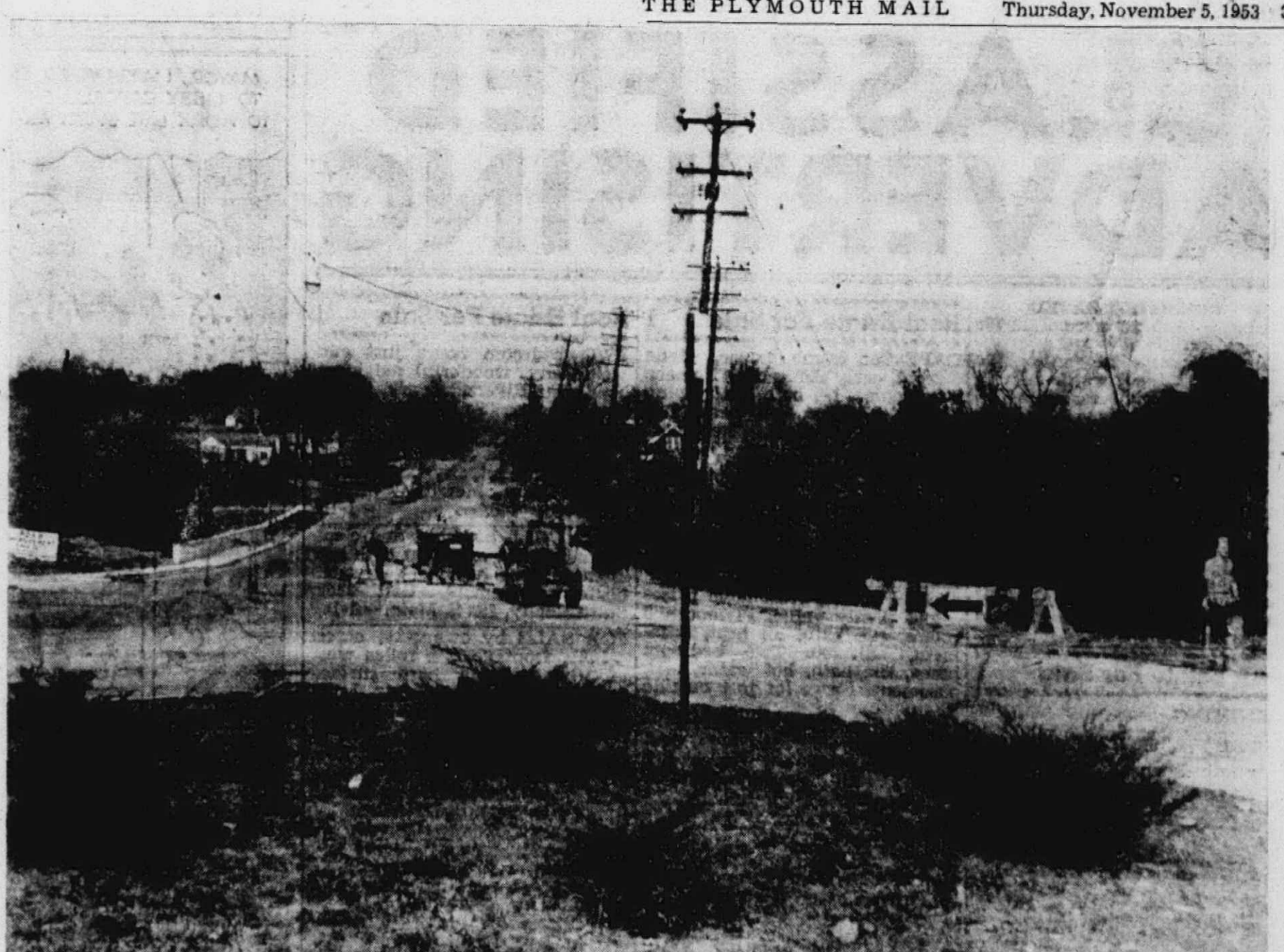
ELIMINATION OF A DANGEROUS INTERSECTION is nearly completed at North Mill street (at right of picture) and Starkweather avenue (left) which join on the north edge of the city to form Northville road. The four-lane bridge across the Rouge river was completed this
