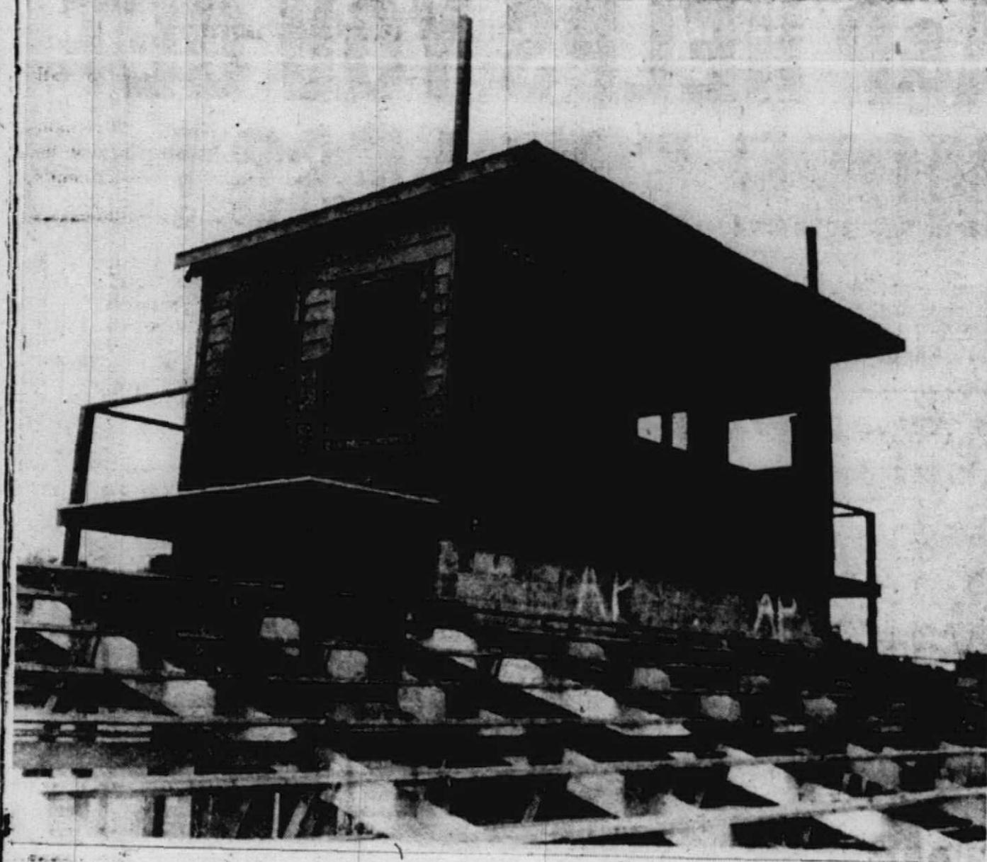
SHOWN ABOVE IS THE RECENTLY completed press box at the Plymouth High school athletic field. Work began on this a year ago and it is now complete with the exception of a few minor details. A new coat of paint was put on a few days ago. The spacious press box will be ready for use this coming football season, and will be a welcome addition to the splendid athletic plant at the high school.
