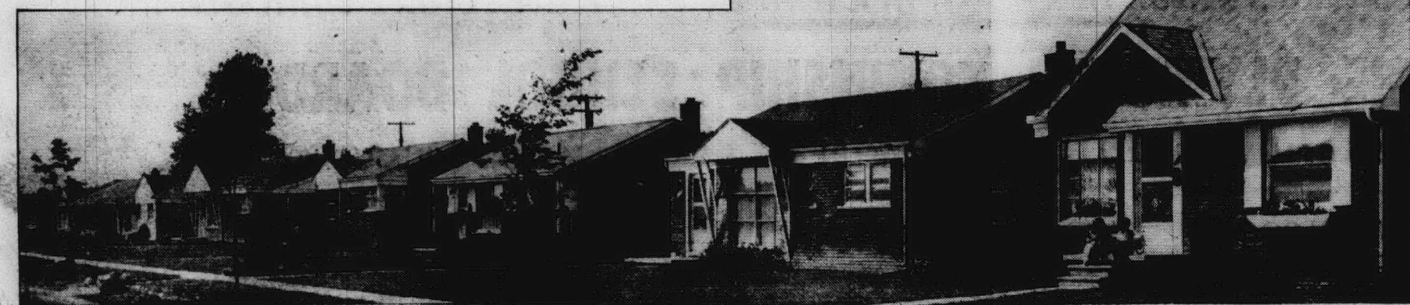
A ROW of recently completed homes at Ross and Lincoln, in Plymouth. New streets have New England names.
