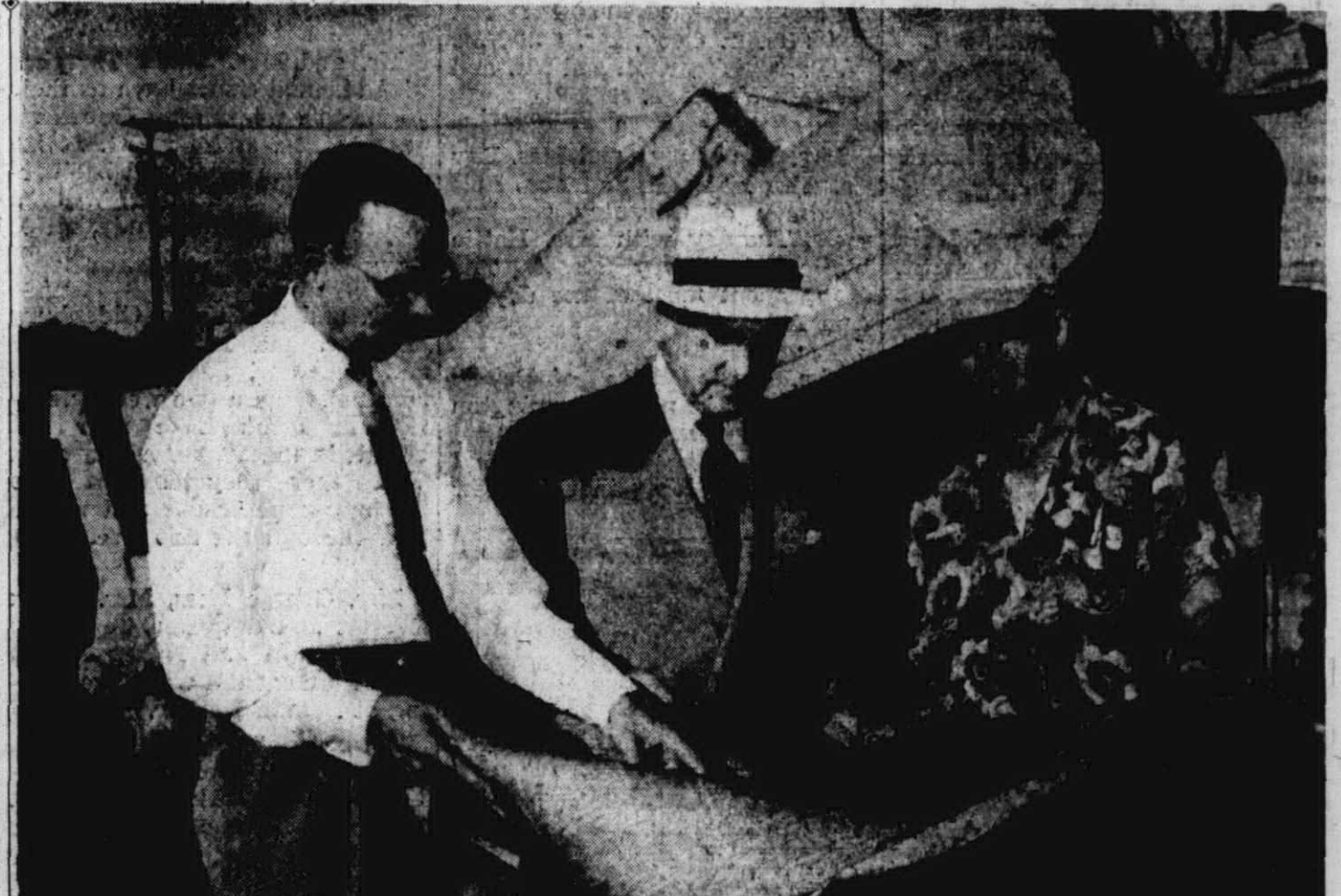
EXAMINING BLUEPRINTS OF DUNN STEEL'S new $500,000 factory-office building are: (left to right) Project Engineer Edward Bergman of the Cunningham-Limp company, general contractors; John G. Spruhan, general manager of the Dunn Steel plant here; and Earl Houghton, construction superintendent. Ground leveling work got underway last week on the seven and one-half acre site located near Hardenberg and Starkweather.
