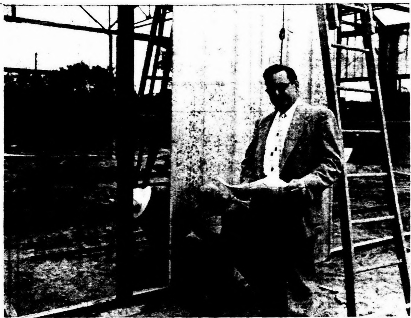
SUPERIOR HEAT TREAT INC. , a new Plymouth industry, is locating at 350 Mill street. Shown in the foreground is James H. Hinckley, president-secretary of the new firm which begins manufacturing here as soon as the first of five divisions making up the $75,000 plant is completed. Employing 10 persons to start, the firm plans to expand to round the clock operations with a labor force of 50. It will heat treat metals to customers' specifications. Hinckley said his company expects to contract extensively with Detroit automotive firms. The divisions shown in the above picture will house two 36-foot car-type furnaces costing more than $100,000.
