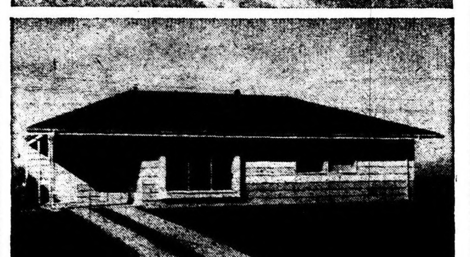
—Photos by Practical Builder Two modern trends in home building, each combining economy and good design, are illustrated in the houses pictured above. One is the inclusion under an extended roof line of a porch that is also a carport, an arrangement that eliminates the cost of a garage and adds spaciousness to the house. The other is the use of asbestos-cement siding shingles as the exterior sidewall finish. Increasingly popular for new home construction, asbestos siding is economical in cost, attractive in appearance and completely incombustible. It is rotproof and weathertight and will last the life of the house without requiring preservative aids. Asbestos siding now is made in many harmonious new colors. In the house in the lower picture colored siding is combined with white for added distinction. The houses, built to sell for around $11,000, are two of 850 in a new Denver, Colo., development.
