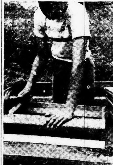
Flats come "knock-down" and are put together with a few nails
