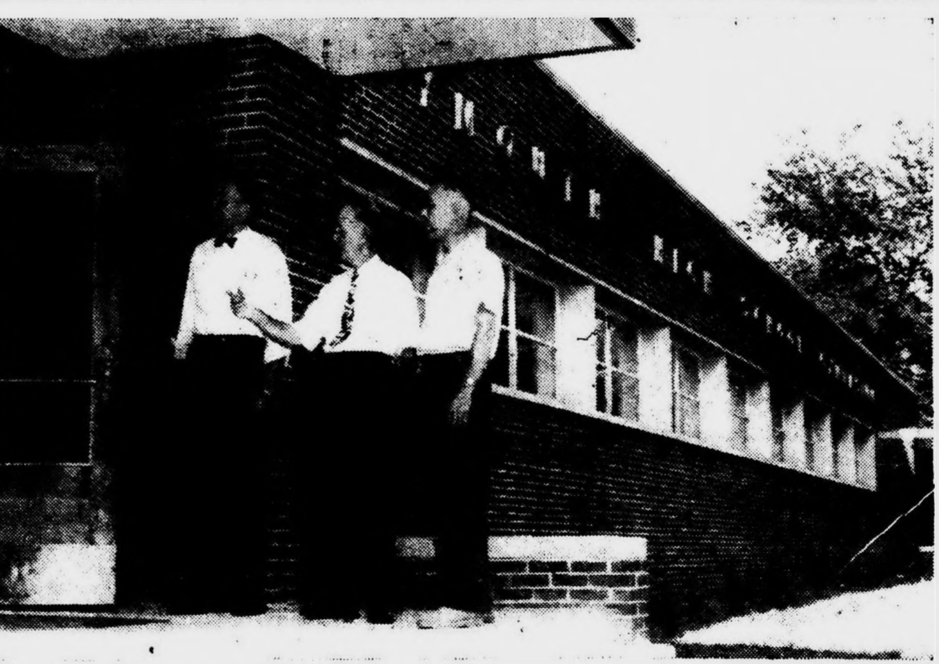
FINAL INSPECTION of Plymouth High School's gymnasium-swimming pool addition is being made by three school officials preparatory to opening the new structure to students starting the school-bound trek, September 4. Shown from l. to r. on the inspection tour are: Superintendent of Schools Russell Isbister, James J. S. Gallimore, President, Board of Education, and Carvel M. Bentley, principal of Plymouth High School.
