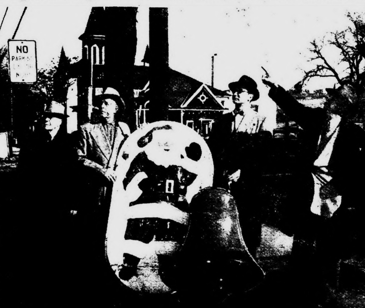
Bert Giles, right, chairman of the Chamber of Commerce city decoration committee, points to where one of the giant ornaments are being strung across Main street in preparation for the Christmas holidays. The work will be completed by the end of this week. Others working on the annual project are, left to right, George A. Smith, chamber secretary; Frank Terry and Marvin Partridge.
