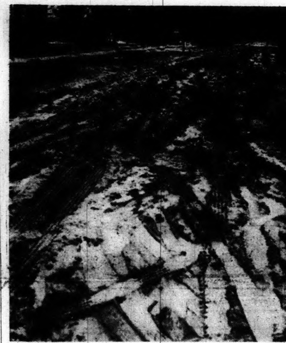
One of the worst streets in the city was Carol avenue, near Harvey. Car owners parked on the nearest paved street and walked to and from their homes, rather than attempt to drive to their garages. Pedestrians find crossing streets like this as hazardous as driving on them.
