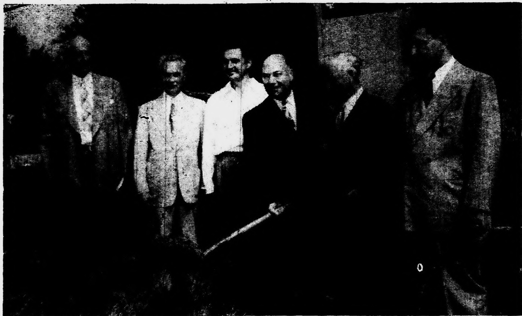
Chamber of Commerce officials watch Mayor William Hartmann turn the first shovel of earth which started a gigantic home building project within the city last weekend. Through the efforts of the Chamber of Commerce the Garling Company of Dearborn started work on ten new homes to be built in the northwest section of the city immediately. Others will follow as soon as these are completed. Participating in the ceremony are left to right, Chamber secretary Charles Hansell, Chamber president Charles Lindstrom, housing committee member Frank Arlen, Mayor William Hartmann, Fred Garling, Sr., and housing committee member Ralph Lorenz.
