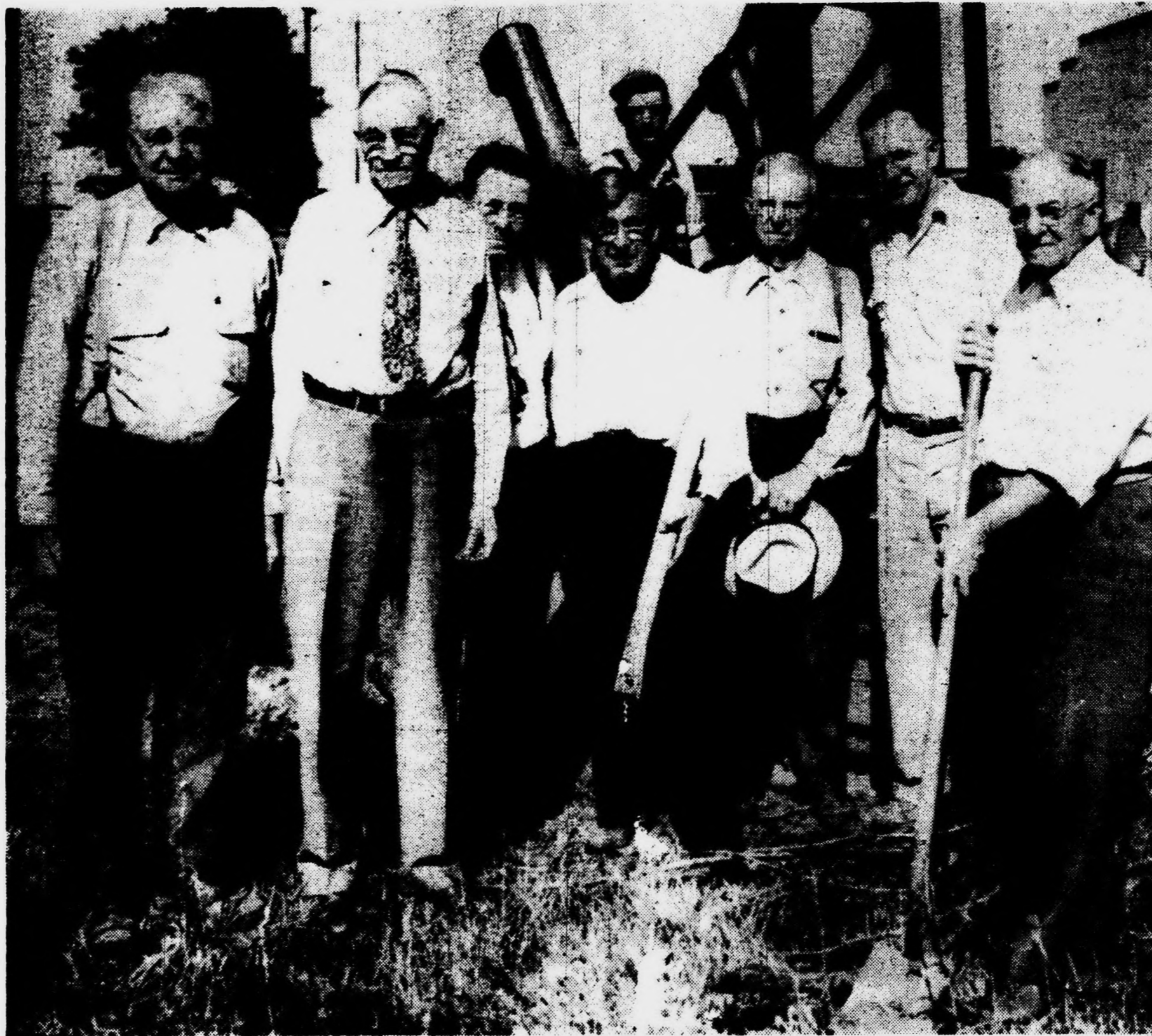
Supervisor Charles H. Rathburn, Jr., was pictured last Saturday ready to turn the first shovelful of dirt on the site of the new township hall to be erected on the north side of Ann Arbor road just east of Lilley road. Grouped in the background to witness the event are left to right, township building inspector Ernest Rossow, township clerk Norman Miller, justice of the peace William Webber, fire chief Roy Jewell, treasurer Sam Spicer, contractor Ernest Burger, supervisor Rathburn and Louis Norman seated on the bulldozer in the rear.
