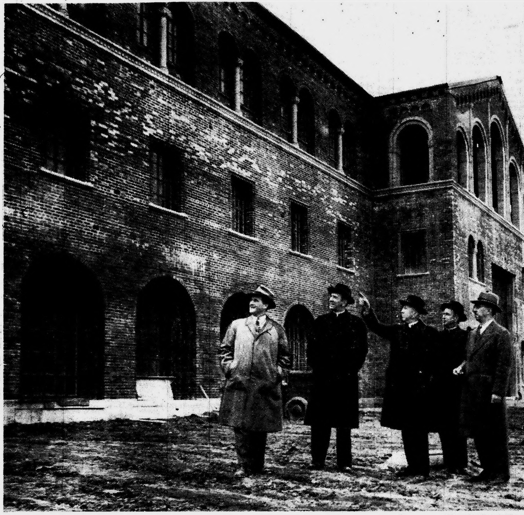
Just a year ago, in April of 1948, ground was broken for St. John's Provincial Seminary, located at Phoenix and Sheldon roads. A recent survey of the building progress was made by those pictured from left to right: Richard Bronnan, the builder; Fr. Andrew P. McEntee, Edward Cardinal Mooney, Fr. John Donovan, and George E. Diehl, the architect. The seminary has been undertaken as a joint project of the five Catholic dioceses of Michigan.
