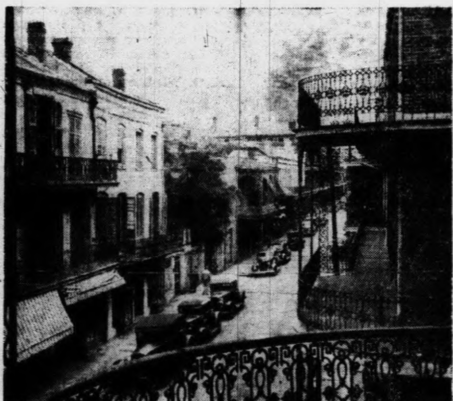
Delicate "iron lace" is a highlight in old New Orleans, and here you have a glimpse of narrow and intriguing Royal street. Originally called Rue Royale-Bourbon, Bienville, founder of the city, changed the name to Rue Royale. Architecture is typically French and Spanish.
