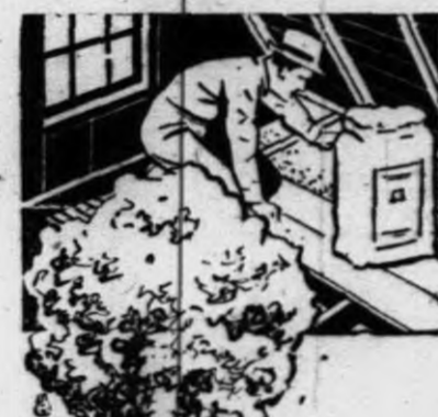
Granulated rock wool for use between ceiling joists or between wall studs.
