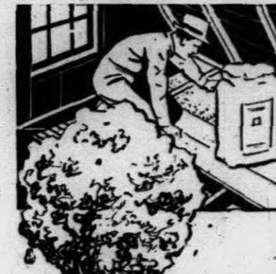
Granulated rock wool for use between ceiling joists or between wall studs.
