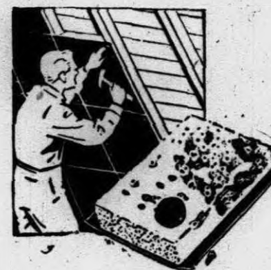
Rock wool batts backed by moisture proof paper for easy application.
