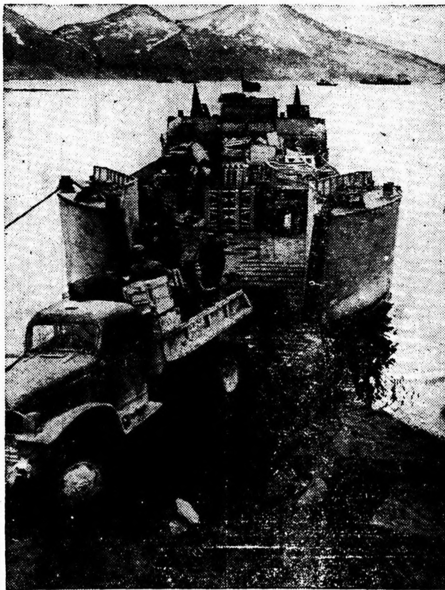
Even as American and Japanese forces on the Aleutian island of Attu blasted away at each other, Seabees of the navy set up bases, supply centers, and generally started military housekeeping. Here a truck carries supplies from a landing boat somewhere along the shoreline.
