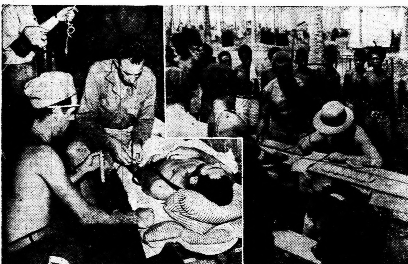
At the site of some of the bitterest fighting of the war, a senior medical officer of the United States naval construction battalion is shown, at left, giving a blood transfusion to a Seabee in a foxhole on Guadalcanal island in the Solomons. At right, several husky natives line up to receive their pay as stevedores. The Seabees—men of the naval construction battalion—are making a base of this island which was wrested from the Japanese after a long battle in which both sides suffered heavy losses in planes, ships, and men.
