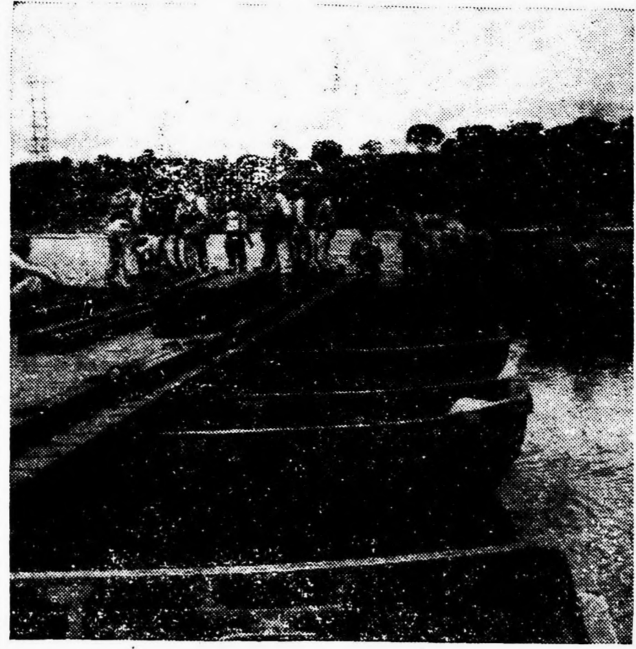
Army engineers in the Canal Zone set what is believed to be an all-time record by spanning a river with a 1,070-foot pontoon bridge in one hour and 40 minutes.
