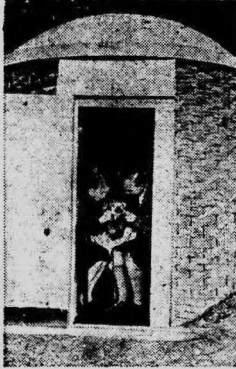
BASKET SHELTER. Running his own air raid precautions program, Henderson Stewart, member of the British parliament, has constructed this new type air raid shelter on the grounds of his home. It consists of a circular wall and roof of concrete. Watlings in a basket-like weave are fastened to the wall on both outside and inside.
