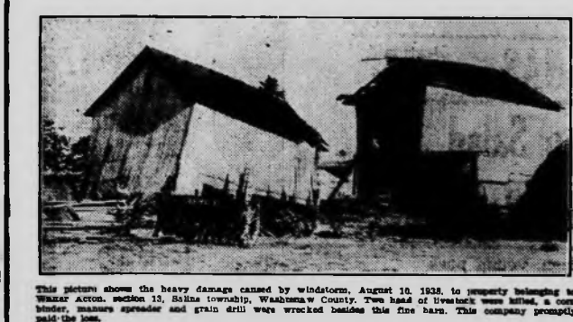
This picture shows the heavy damage caused by windstorm, August 10, 1938, to property belonging to Wazlar Acton, section 13, Saline township, Washtenaw County. Two head of livestock were killed, a corn binder, manure spreader and grain drill were wrecked besides this fine barn. This company promptly paid the loss.
