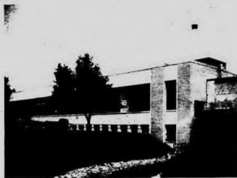
The new Northville plant, showing the waterwheel that provides part of the power. Motor valves are made here.
