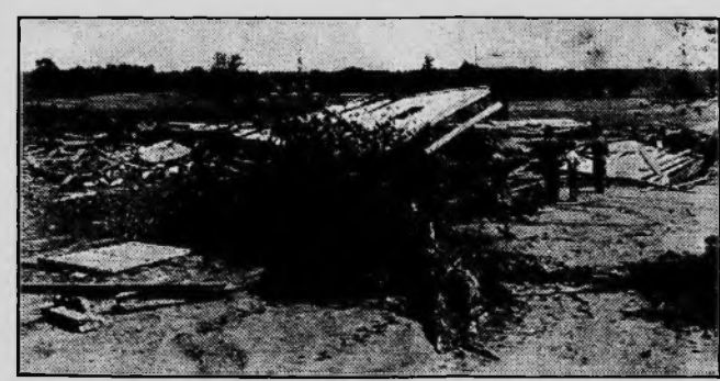
The above picture shows the damage done to property belonging to Flande R. Cleveland, Somerset township, Hillsdale county, by a windstorm which swept through that part of the State June 20, 1887. Two sets of buildings were partly covered with windstorm insurance. The total loss paid by this company was $3,548.18. These buildings were on sections 35 and 38. It pays to have property well covered with windstorm insurance.
