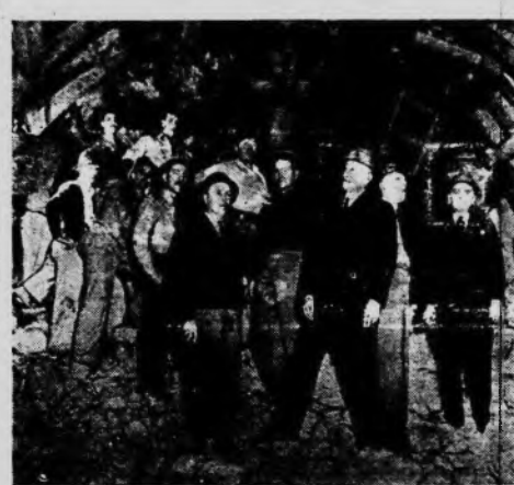
Interior of East Coachella tunnel in California, the longest tunnel in the world, after a charge of dynamite tore out the last barrier of rock and holed-through the 242-mile-long bore. The tunnel will carry water from the Colorado river to Los Angeles.
