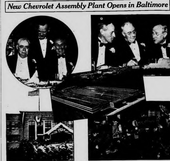
Governmental, state and civic officials joined with the principal executives of General Motors Corporation in the formal opening of the new 80,000-car-a-year Chevrolet assembly plant in Baltimore recently. The new plant (center) was dedicated with impressive ceremonies (lower left), and Chevrolet, Fisher Body and General Motors officials were guests of the Baltimore Association of Commerce at a formal banquet in the evening. W. E. Holler, vice-president of the Baltimore Association of Commerce, is shown (standing) with Maryland's Governor, H. W. Nice, and Alfred P. Sloan, Jr., president of General Motors (upper left). M. E. Coyle, president and general manager of Chevrolet, is pictured in the upper right photo with Senator Millard Tydings (left) and Mayor H. W. Jackson, of Baltimore (right). Lower right shows the first motor car built in that city.
