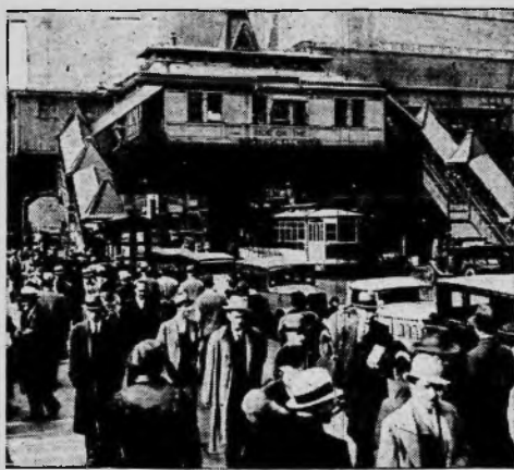
HERE is a view of the most dangerous crossing in New York city, the intersection of Sixth avenue and Forty-second street. A police survey has given it its bad reputation, showing that during 1933 forty six persons were injured and one killed in traffic accidents there.
