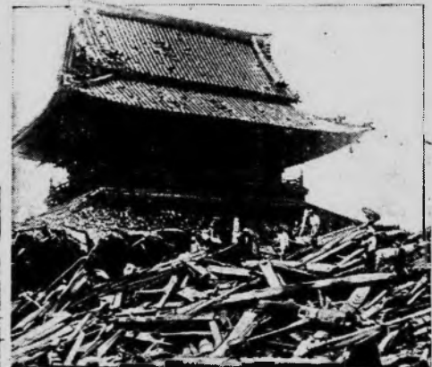
AMONG the many buildings destroyed by the recent typhoon in Japan was the Tennoji, a famous shrine at Osaka which was erected about fifteen hundred years ago. It was considered by the Japanese one of their national treasures. The photograph shows the shrine after its collapse.
