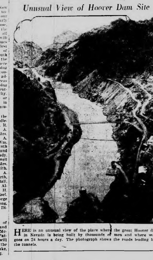
HERE is an unusual view of the place where the great Hoover dam in Nevada is being built by thousands of men and where work goes on 24 hours a day.
