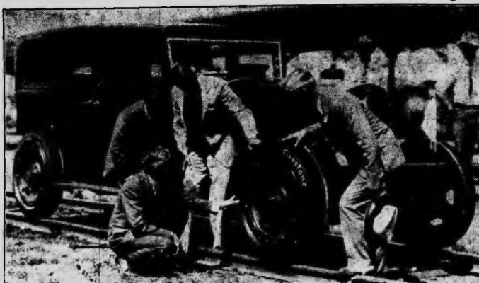
Harvey S. Firestone (left foreground) stands the new Firestone rail tires in perfect condition after they had enabled an automobile running on railroad tracks to set a record between Miami and Jacksonville, Florida.
