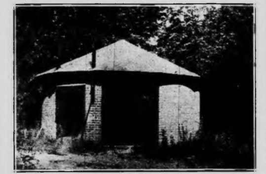
This circular structure standing in a small open space in the woods houses the electric pumps of the Plymouth water system.
