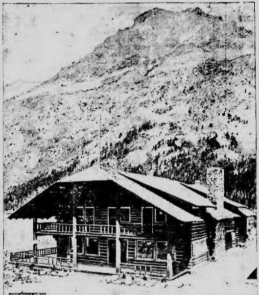
Two Medicine, Lake Chalet, where President Hoover's office work will be done during his stay in Glacier National park. This building will also serve as the dining hall for the Presidential party. Rising Wolf mountain can be seen in the background.
