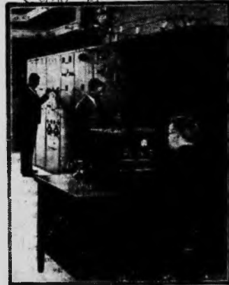
Power Panel and Control Turret
