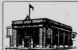
The Bank On The Corner
