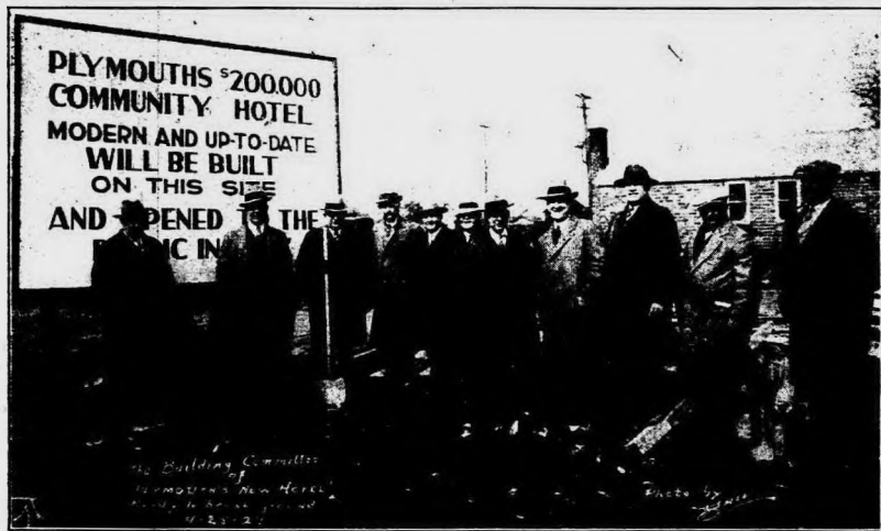
The first spadeful of earth was turned for the new hotel on April 25, this year, when the corporation building committee, architects and contractors assembled for the ceremony. Reading from left to right, the picture shows: Mr. Knox of architect's office; J. H. Wettlauffer of Stibhard Construction Co., contractors and builders; F. D. Schrader, who turned the first earth; Carl Shear, John Larkins, E. K. Bennett, E. O. Huston, E. B. Wilhelm, architect, Paul Wiedman, Edward Gayde and Frank Rambo.
