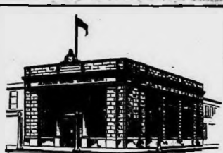
The Bank on the Corner
