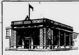
The Bank on the Corner
