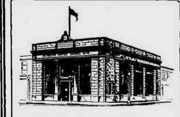
The Bank on the Corner
