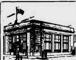
The Bank on the Corner
