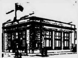
The Bank on the Corner
