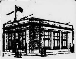
The Bank on the Corner
