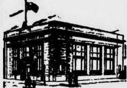
The Bank on the Corner
