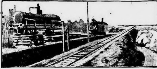
Novel Makeshift Water Tank Improved to Serve Railroad Engines Employed during Construction of a Canadian Electric Line.
