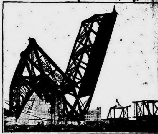
Huge Three-Track One-Leaf Swing Over the North Branch of the Chicago River, Replacing the Lifting Structure Which is Seen at the Right, Resting, Bisected, on Its Center Pier.
