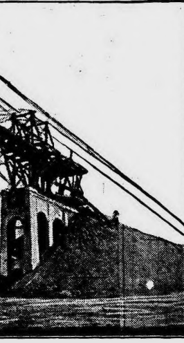
The Wooden Cantilever Traveler in Use Beginning the Erection of the Viaduct at Lewistown, Mont.
