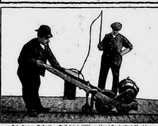
Grinding a Defective Rail-Joint With a Hand-Controlled Machine.
