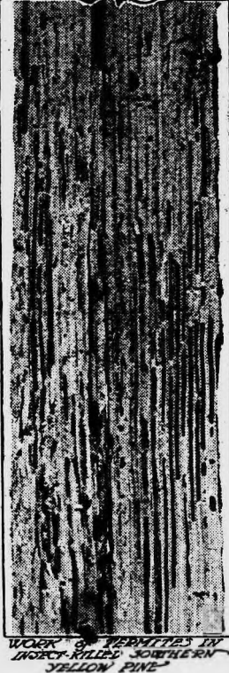
WORK OF TERMITES IN WOODS. SHEDS SOUTHERN YELLOW PINE.
